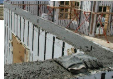
ARXX ICF stack easily and quickly to create a monolithic, energy-efficient, structurally tough wall.
